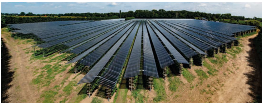
Figure 4-2 Light transmission achieved using transparent panels application. SolarPower Europe, 2020
